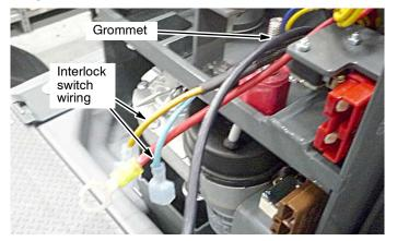
5. Reconnect the interlock switch wires to the new interlock switch as shown.
